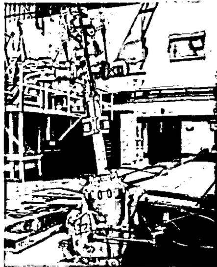
The first of two Bell XV-3s rolled out of the Hurst, Texas plant in 1955 (left). An electric motor moved the rotors from vertical to horizontal in 20 seconds (above).
